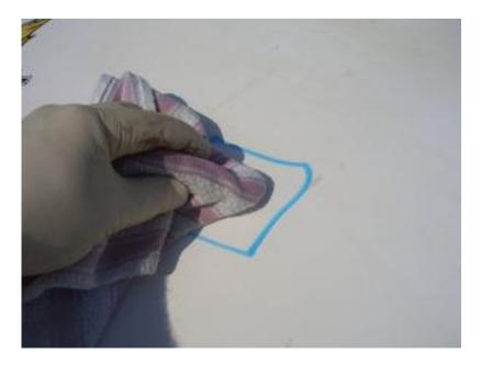
Clean off the sanded area with alcohol again, to make sure there's no grease on the surface.
