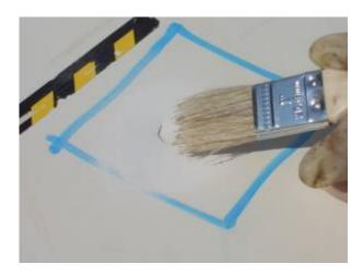
With a clean brush, wet the board surface around the hole with resin/hardener mix. This ensures that the epoxy will get a good grip on the surface of the board.
