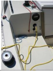
Why: The boat moves around. If the cord is wrapped tightly around something, the boat will put tension on the cord and pull out the clamps that hold the cord to the dock.
