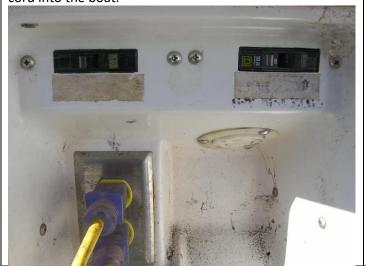
Do: Make sure the power is off before plugging in the boat and the power is switched on after the boat is put away.
