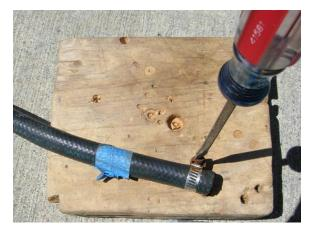
Cut through the hose approximately <sup>3</sup>/<sub>4</sub> of an inch (2 cm) from the end. If you hit the broken piece of the connector, make cuts around the hose until you can remove the broken piece.
